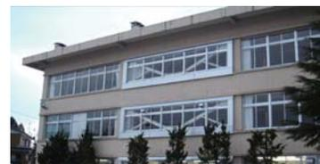
An elementary school that has been reinforced against earthquakes with steel braces
