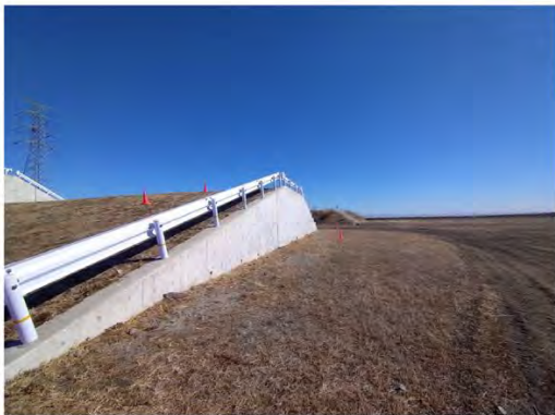
(Fig.3) Picture of slope and some feature points on the course
