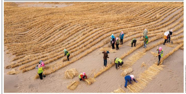
Workers plant straw barriers in desert areas in northwest China's Gansu province to stop sand from spreading, aiding afforestation.
