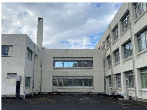
③ B・C 棟間
