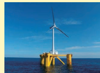
Floating offshore wind-power generation facility
