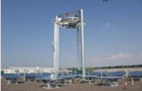
**Tower Type Solar Thermal Power Generation Technology Operation Test Plant (Abu Dhabi, UAE)**
