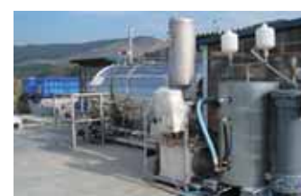
Picture of the entire biomass energy recovery system
