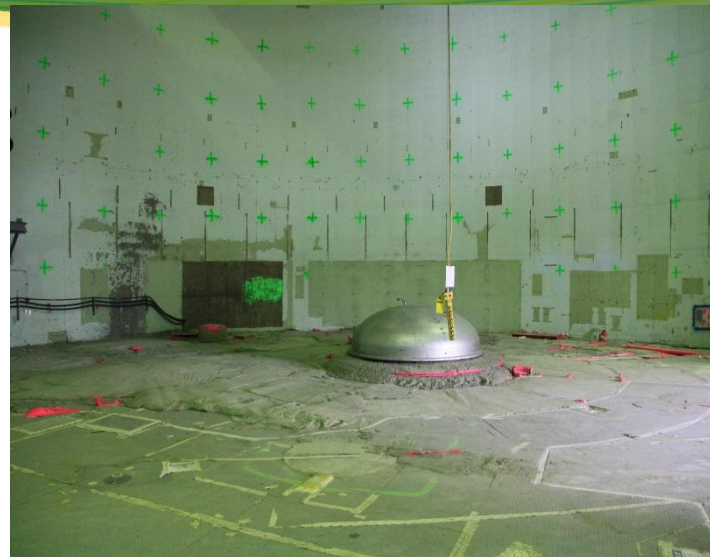
Reactor is now Entombed with Grout
