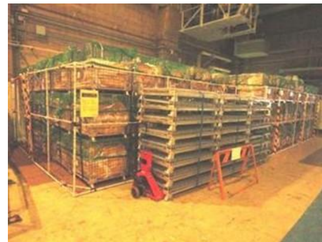
Fugen's waste from dismantling awaiting measurements for clearance
