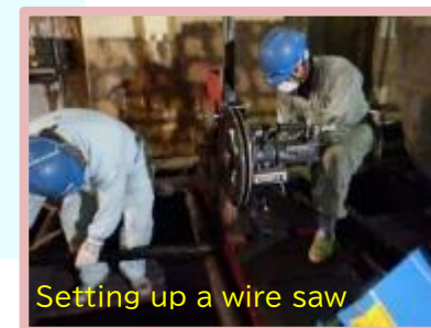
Cutting coolant pipes simultaneously using a wire saw
