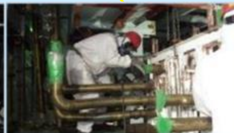
Cutting inlet pipes
