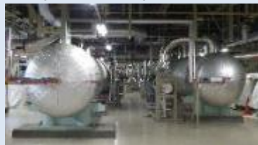
High-pressure feedwater-heaters 1 and 2 (before dismantling/removal)
