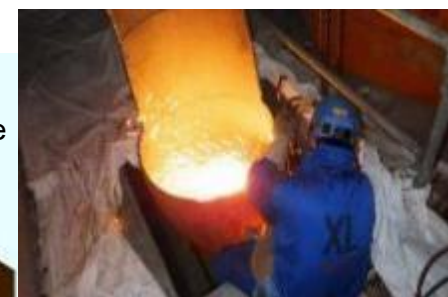
Cutting a high-pressure turbine exhaust pipe
