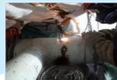
Cutting ECCS pipes
