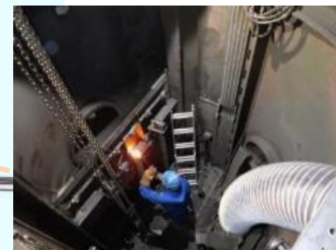
Cutting the internal structure of a moisture separator
