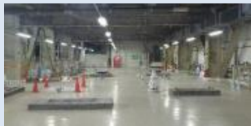
High-pressure feedwater-heaters 1 and 2 (after dismantling/removal)
