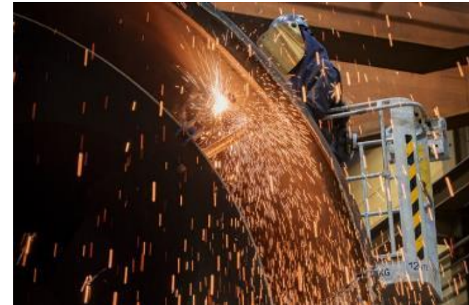
Segmentation (hot cutting)
