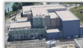
ICEDA Conditionning and interim storage facility for IL waste long life Start of operation : 2020
