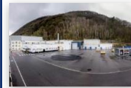
Chooz A PWR 1967-1991 Decommissioning decree: 2007
