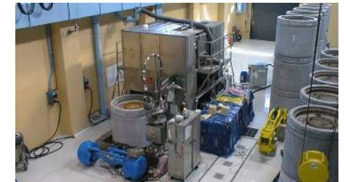
Deployment of mobile machines to condition legacy waste / substances: sludge, boron, resins...
