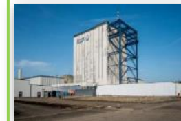
Bugey UNGG 1972-1994 Decommissioning decree: 2008
