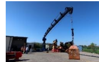
Supply and set up of the main auxiliary handling system for SG extraction Also use for
