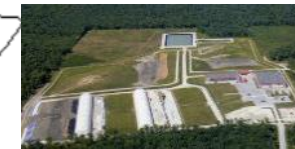
CIREs Waste repository (VLL waste) Start of operation : 2003
