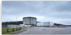
Brennilis HWR 1967-1985 Decommissioning decree: 2011
