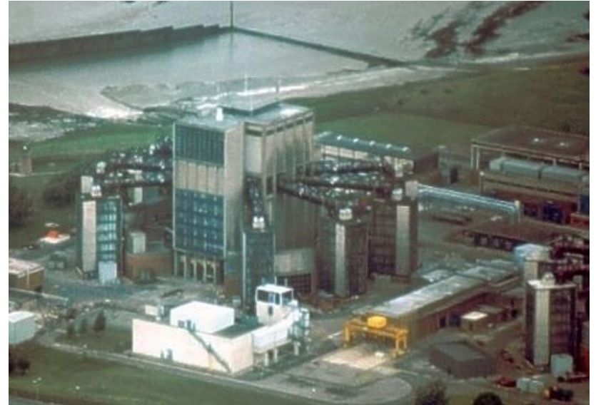
Berkeley Power Station prior to decommissioning
