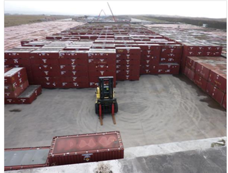
Low Level Waste Repository – Capacity Challenge
