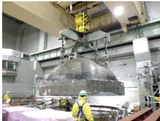
Removing the pressure vessel top lid
