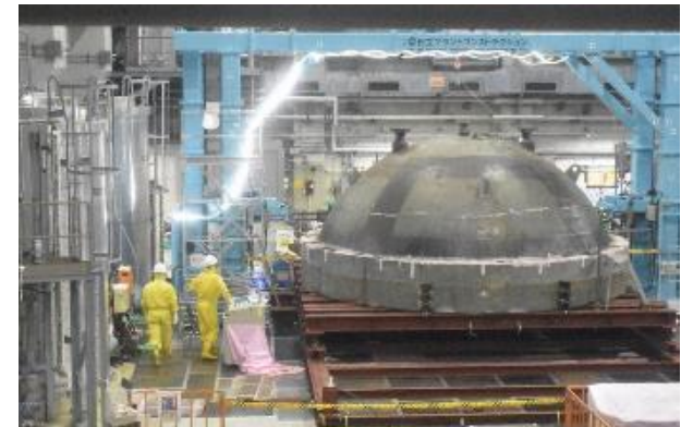
Cutting work using a large band saw
