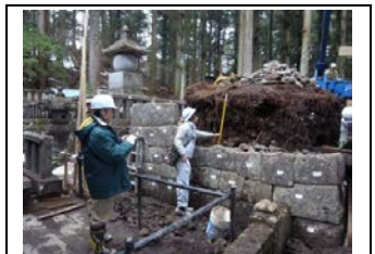
Restoration work for Jigendo Pagoda at Nikko Rinnoji Temple (photo courtesy of Nikko Cultural Assets Association for the Preservation of Shrines and Temples)
