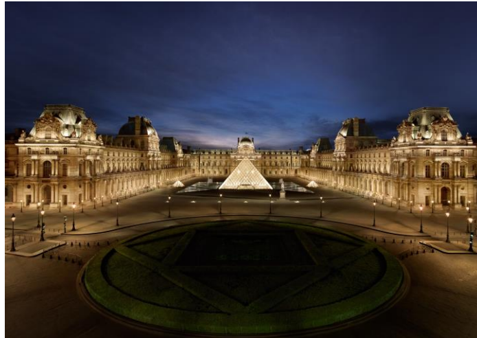
Louvre Museum Lighting Refurbishment Project
