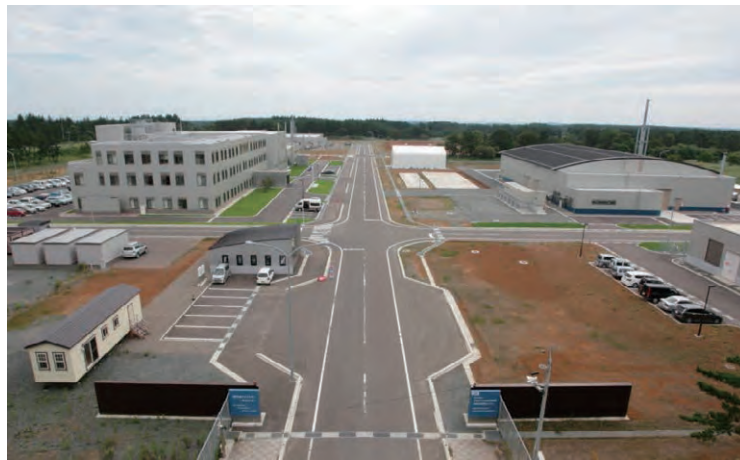
International Fusion Energy Research Center (Rokkasho Village, Aomori Pref.) Courtesy of JAEA
