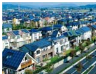
Photovoltaic power generation system installation in test site area ("Pal Town Josai-no-Mori," Ota-shi, Gunma)
