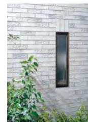
Self-cleaning tiles using photocatalysts Photo: TOTO Ltd.
