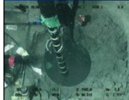
Construction of Installation hole for seismometer
