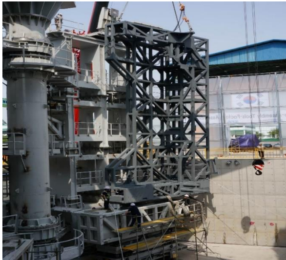
FAT with a load of the VVTS OB Sector Frame
