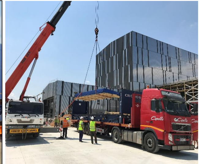
1st delivery package arrived at IO Site on 23 rd June
