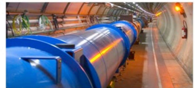
Continuous magnet line installed in the 27 km LHC tunnel, 2006
