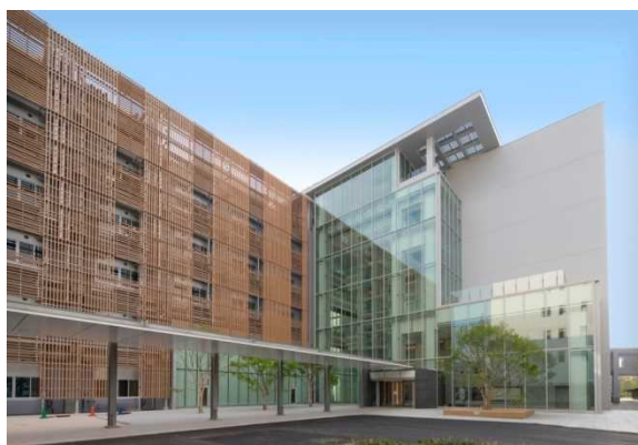
MANA building in NIMS, Tsukuba
