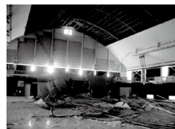
A Ceiling of a gymnasium collapsed partially due to the Niigata-Chuetsu Earthquake (Unuma City, Niigata Prefecture)
