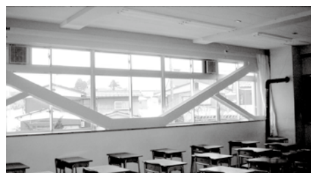
Appearance of a school building reinforced to resist earthquakes (Tokamachi City, Niigata Prefecture)
