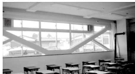
Appearance of a school building reinforced to resist earthquakes (Tokamachi City, Niigata Prefecture)
