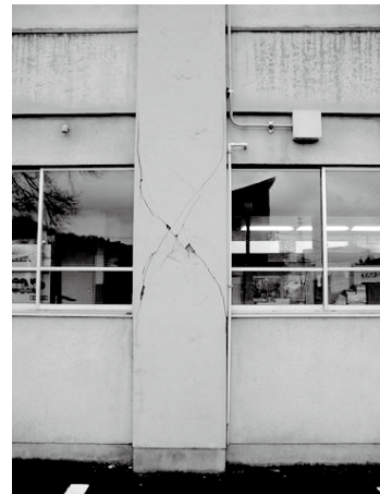
A pillar of a school building cracked by the Niigata-Chuetsu Earthquake. (Ojiya City, Niigata Prefecture)
