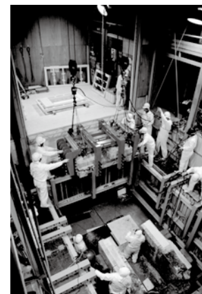
The hauling of the ceiling stones (28 May 2007)
